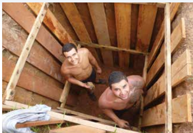
Jaymin Cameron (L) and Jameson Pulelisi constructing a pit toilet in an Amazon village.
